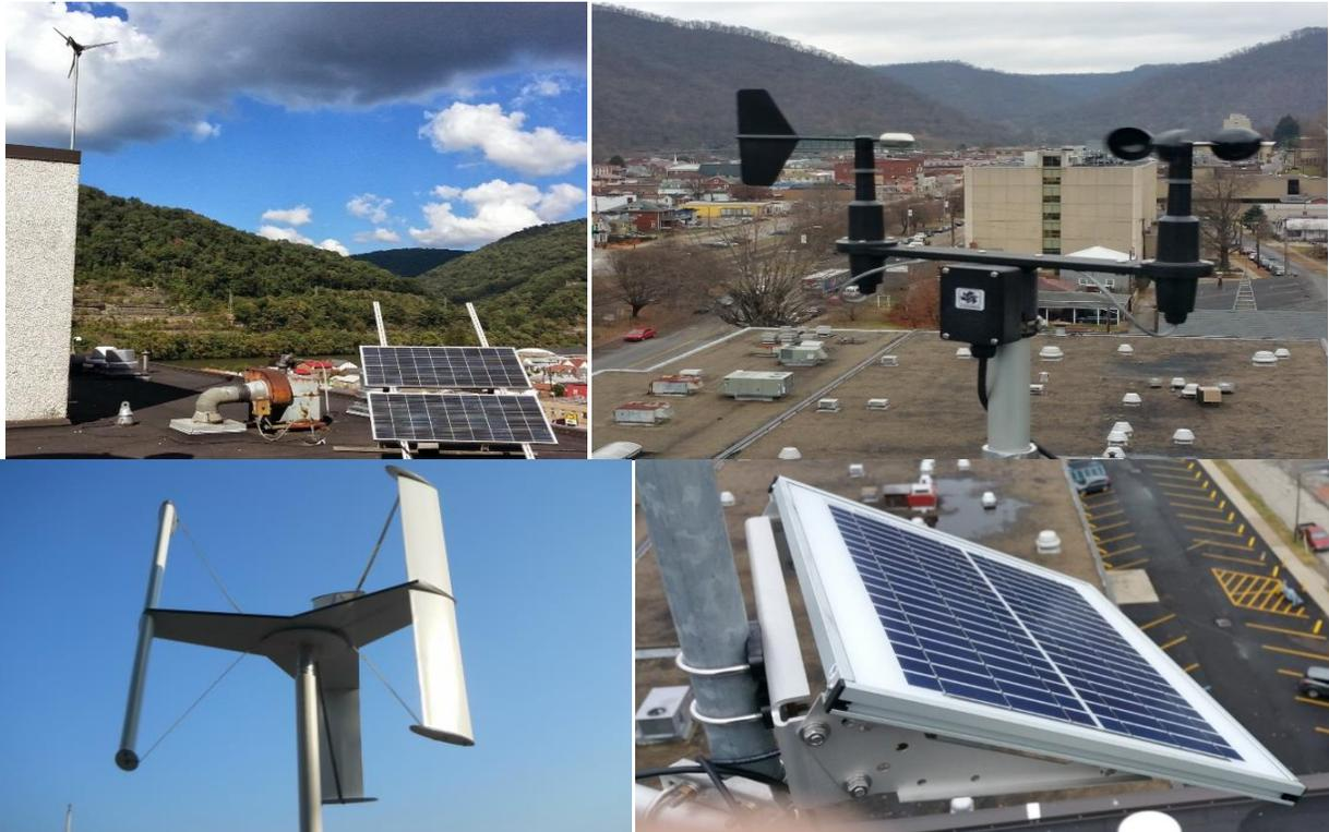
Figure 1: Residential wind turbines (both horizontal and vertical wind turbines), solar PV units, and weather station installed on the roof of the engineering building
