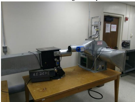
Figure 3: VFD and Centrifugal Fan Installation
