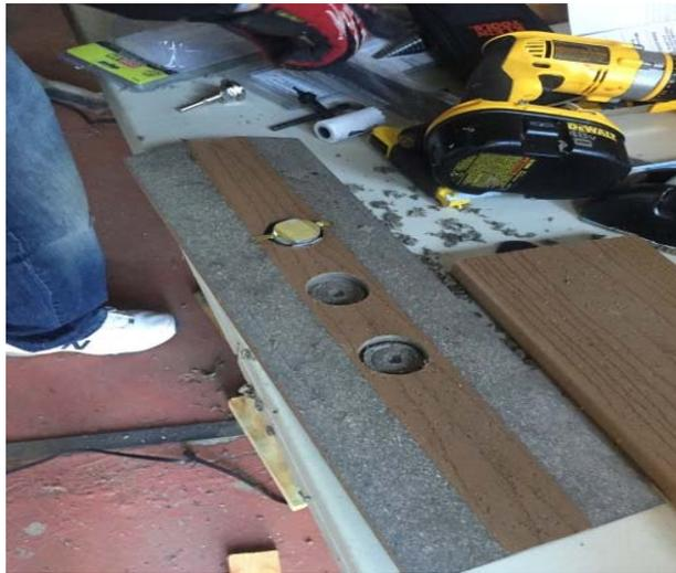
Figure 3: Board Construction
